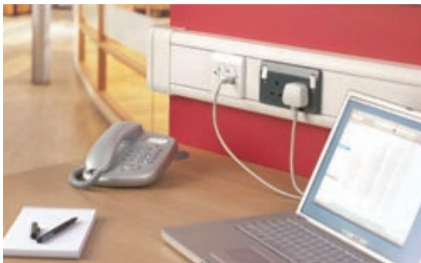
The design consideration 4.29 also requires individual switches on multiple socket outlets and panels to be 'well separated' to prevent inadvertent operation. However, no guidance is given as to the dimensions of the required separation. When installing twin socket outlets, those with outboard switches should be specified.
